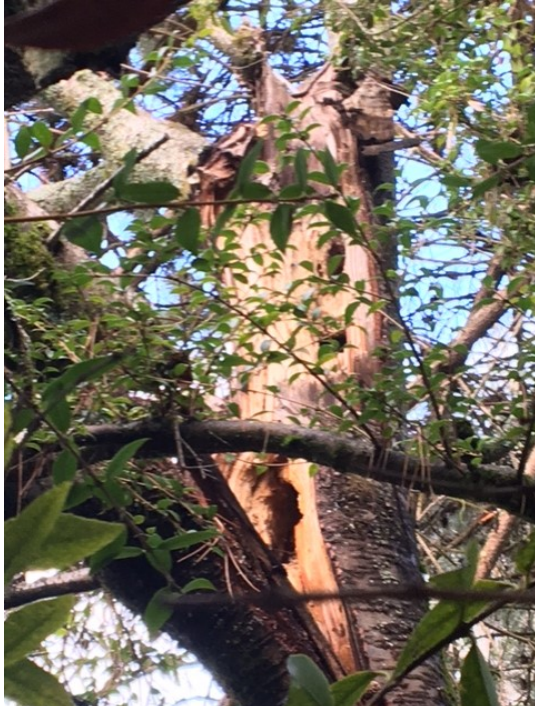
Photo 1. Large broken and hanging tree Top of Tree #5.
